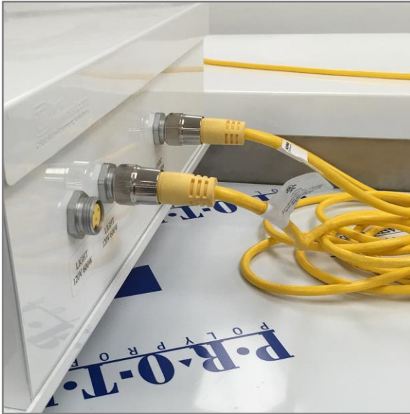
Figure 13. PDM connections for light fixtures
