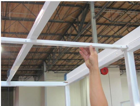
Figure 8. Position the Support Bar below the joists
