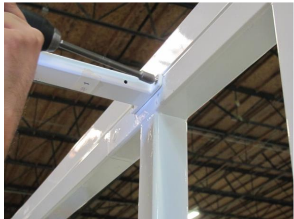
Figure 9. Fasten the support bar to the frame
