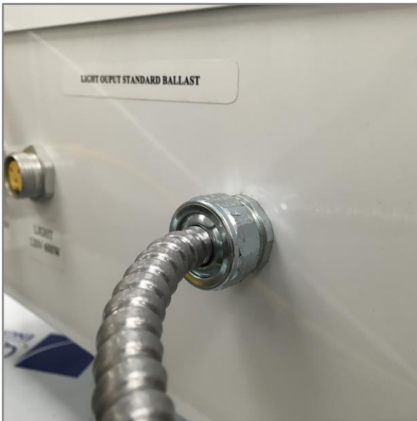
Figure 15. Wiring inlet for outlets on standard PDMs
