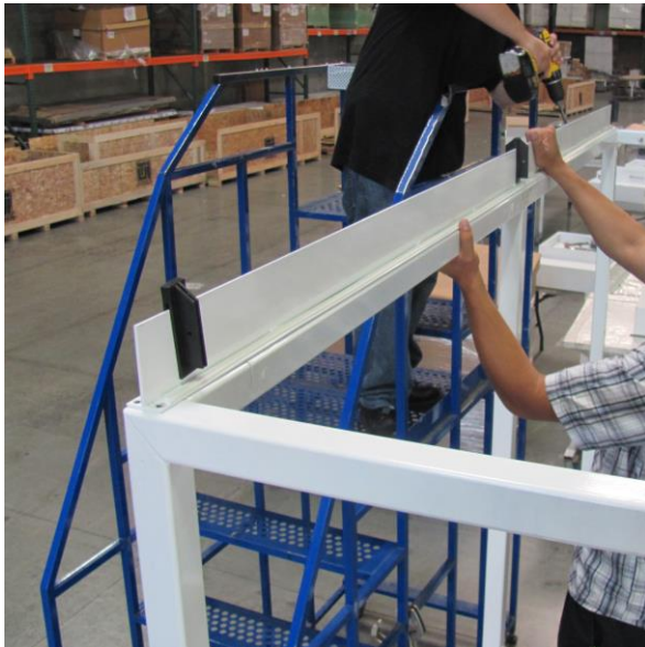
Figure 4. First and last joists rest fully on the frame
