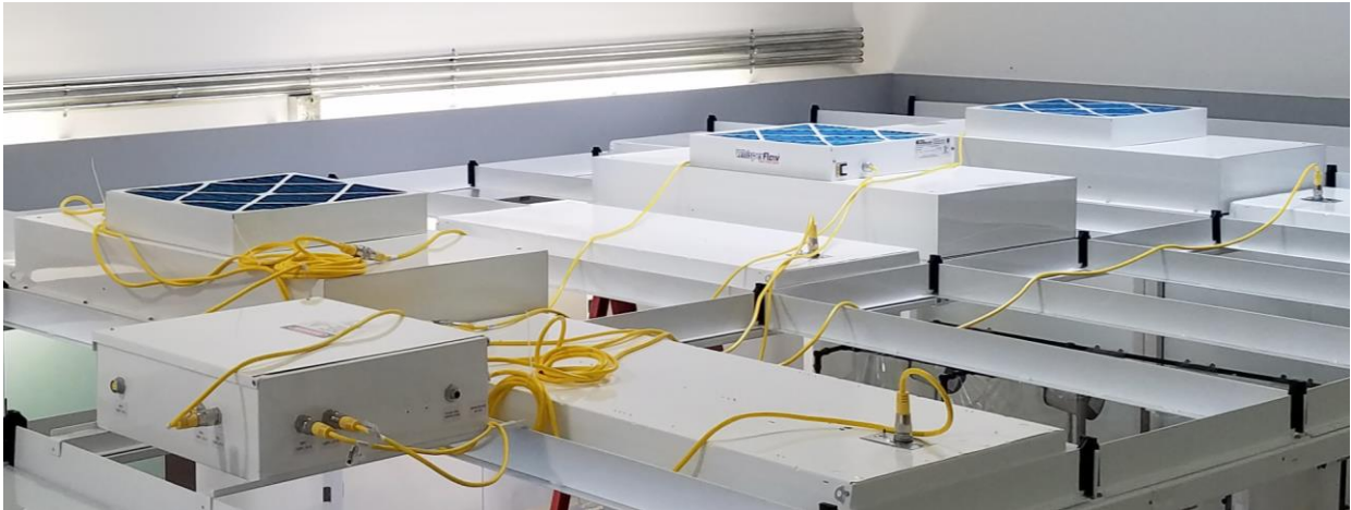
Figure 10. Typical ceiling grid during installation with PDM, three FFUs, and three Fluorescent Light Fixtures visible (blank ceiling tiles have not been installed yet)
