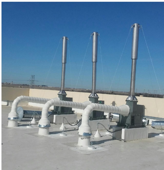
Typical Class II BSC Exhaust System
